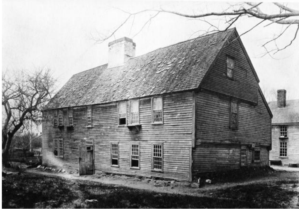
The Whipple House on Saltonstall Street before restoration
