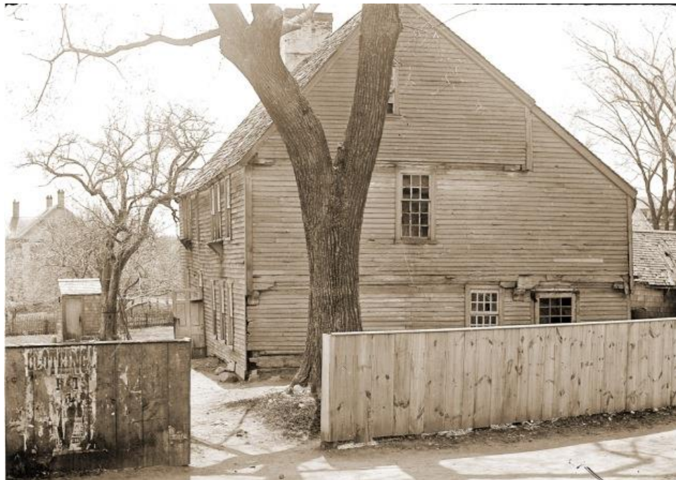
The Whipple House during restoration on Saltonstall Street. Typical of First Period houses, it faced south to take advantage of warmth from the sun.
