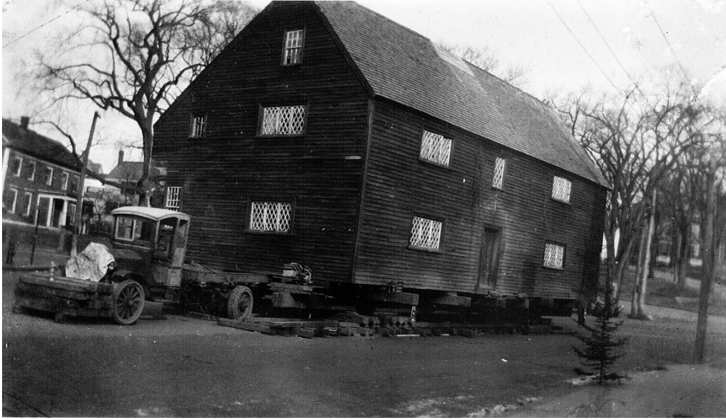
The Whipple House being moved, at the intersection of Market St. and Market Square
